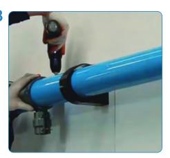
• Tighten the bolt to complete assembly.
