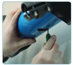
• Remove debris and deburr cut edges.
