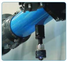
Apply steady pressure until the hole saw bit has completely entered the pipe.
