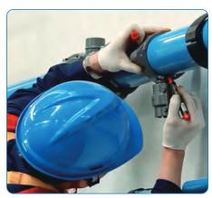
• Mark the pipe where the hole for the quick drop connector will be installed.
