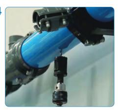
Hold the drill perpendicular to the pipe with the drill bit in the center of the mark placed on the pipe. 05
