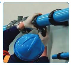
• The quick drop connector easily aligns into the drilled hole.
